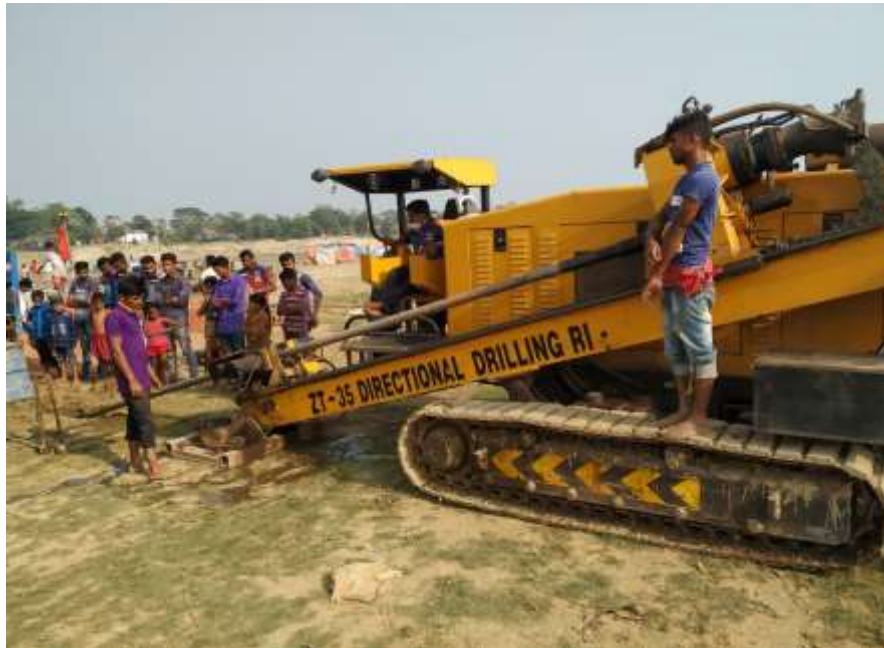
Figure 2. Horizontal Directional Drilling (HDD) Work
