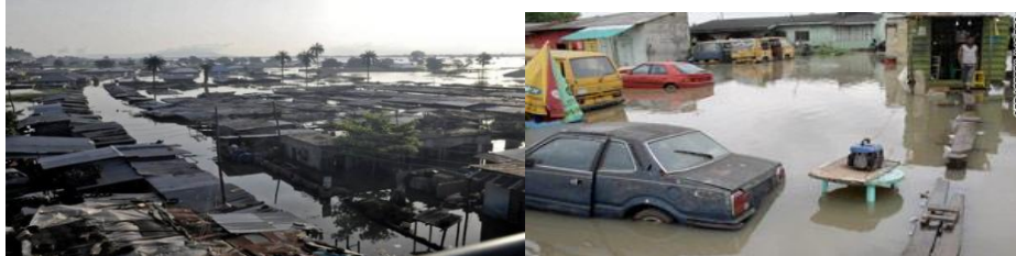
Figure 7: Images of Flood Disaster in Nigeria
